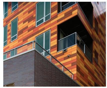
Available in any color, with the ability to match colors of your choice without expensive up charges – Dri-Design Painted Aluminum Panels offer the ultimate design flexibility for exterior and interior applications. Panels are painted using industry leading Fluoropolymer based paints for long lasting finish durability, while our finishers use a 100% air capture system to destroy the VOCs produced, so there is no adverse environmental impact.
