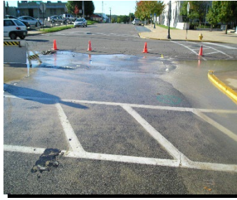
Leak surfacing at intersection
